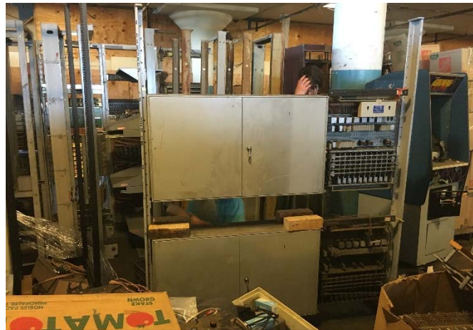
Senders mounted to framework in Jim's warehouse
