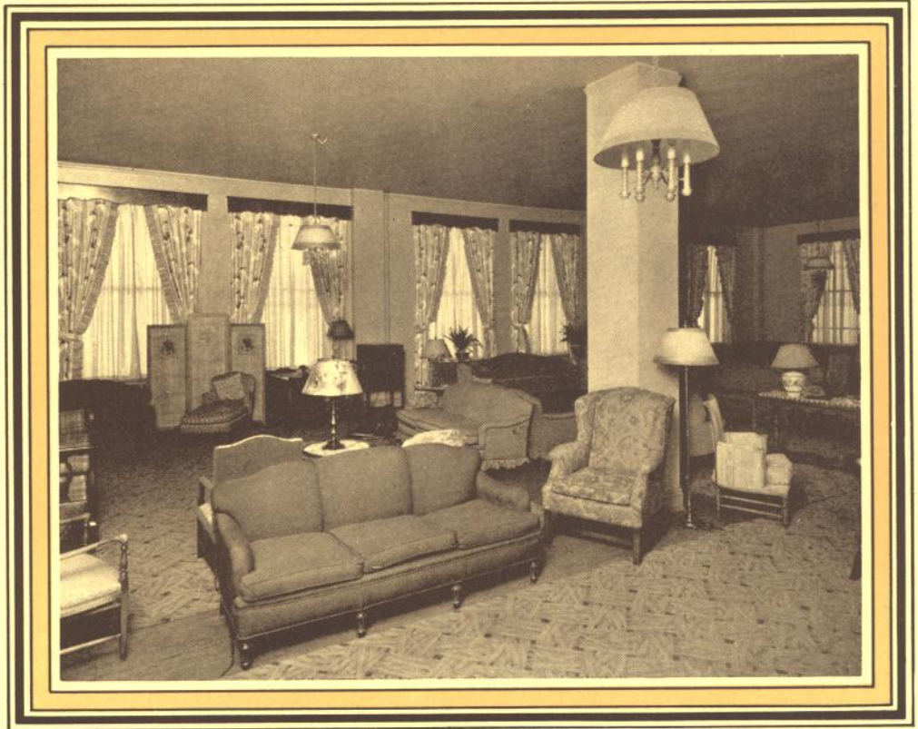
Operators' Rest Room. In contrast to the business-like concentration of the operating room.
