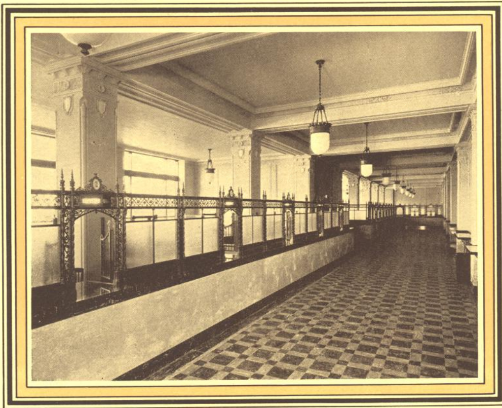
A view of one side of the business office, designed for the convenience of the public.
