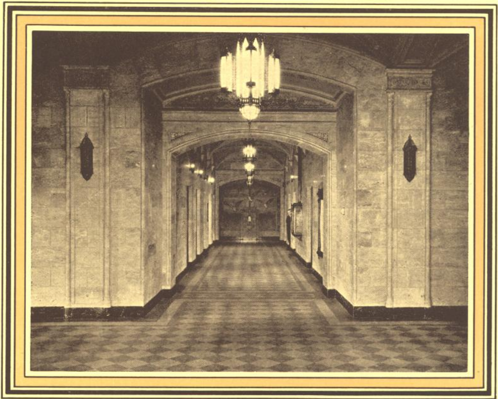
The Elevator Lobby with walls of Colorado Travertine. The elevators are of the latest automatic signal control type and travel nearly twelve feet a second.
