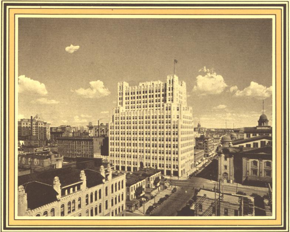
A view of completed building from Fourteenth and Arapahoe Streets. Almost entirely a product of Colorado materials and workmanship.
