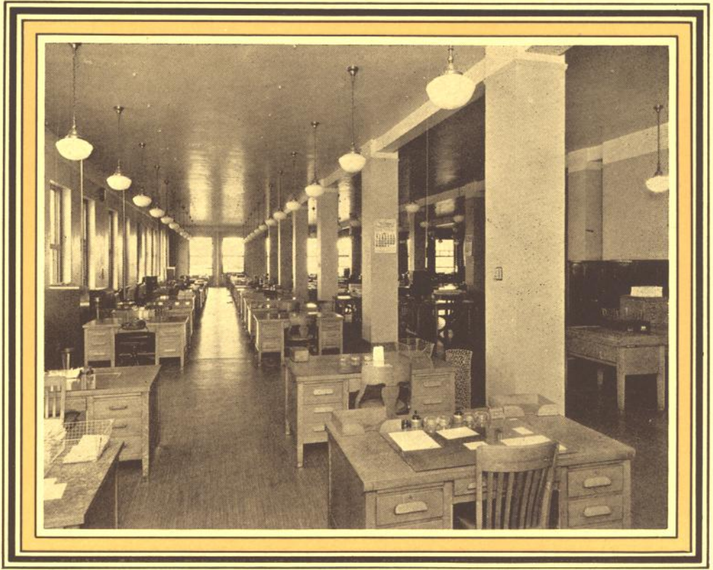
A typical office, the Colorado Accounting Department. Tints and fixtures were carefully selected; heating and ventilating devices are of the most modern type.
